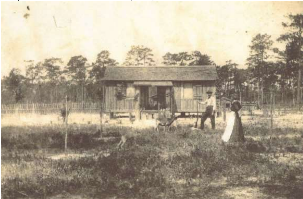
Finley B. Click and his wife Maggie, outside his second cabin, Ethel, 1912. The airway through the cabin probably separated the parent's bedroom from the main room where the children would have slept. Behind the cabin is a fenced area for the animals and to the right of the cabin an outside shed or animal coop.
