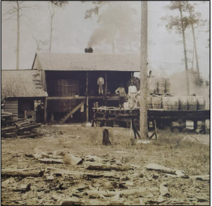
Turpentine still (Source: WSSP)
