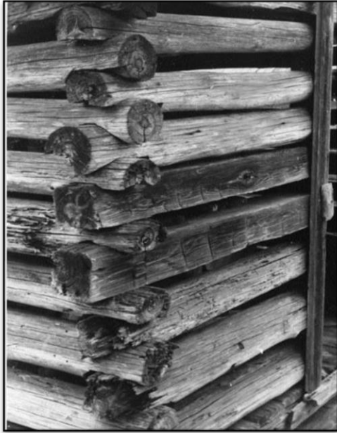
Cabin construction using notched log. Source: Florida Memory
