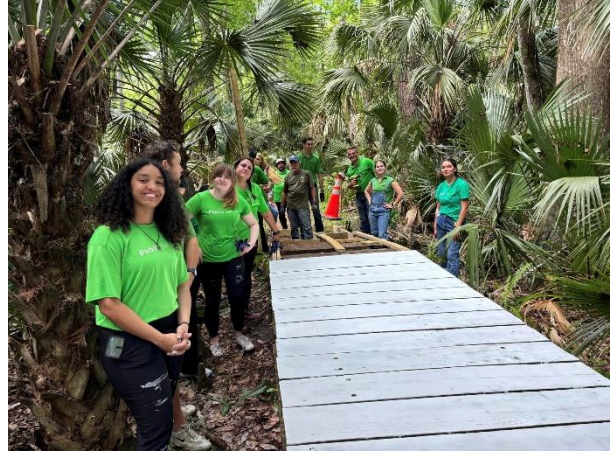
Repairing the boardwalk
